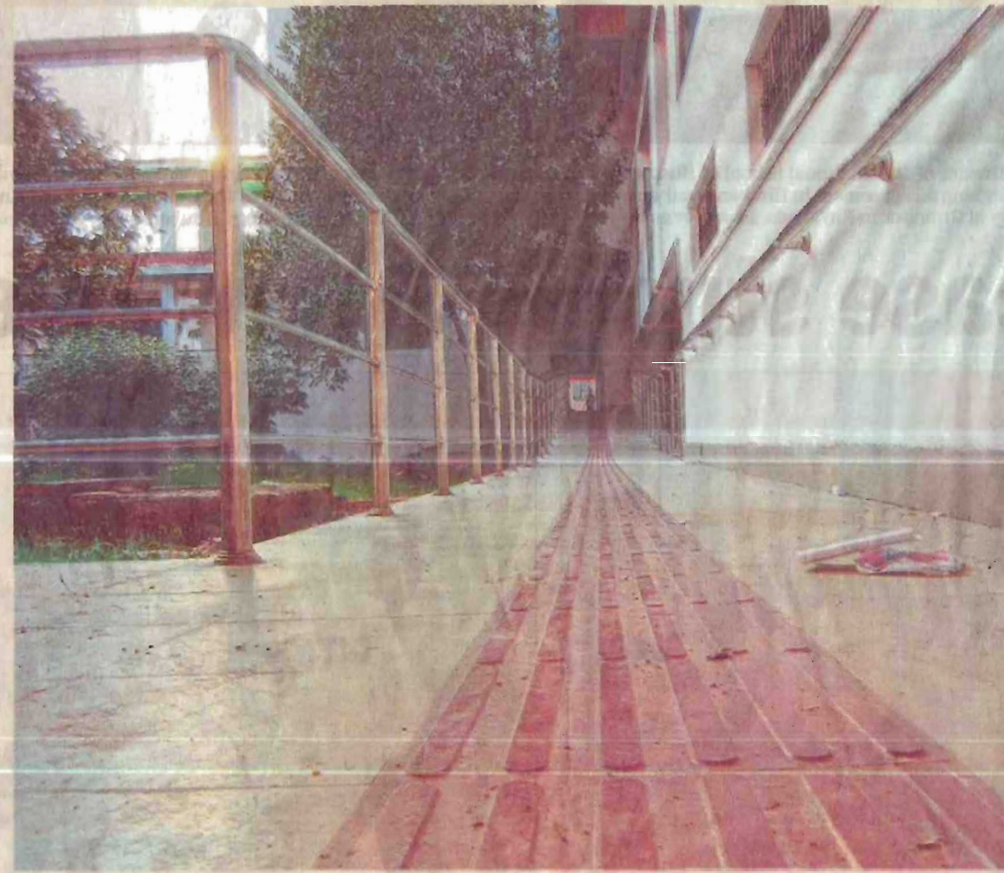
A ramp with guiding tiles at Nirman Soudha (office of the chief engineer, public works department) in Bhubaneswar. Picture by Ashwinee Patil
